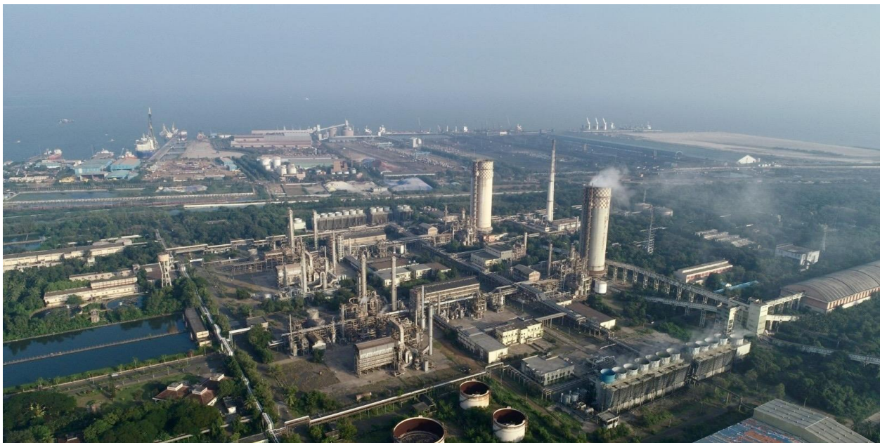
Ammonia production facility and port infrastructure on East coast of India
